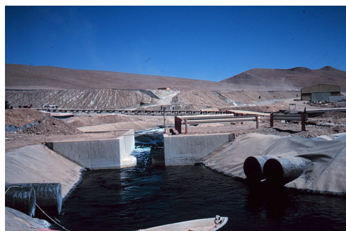
Fig. 4. Heap bioleaching for copper recovery in Quebrada Blanca, Chile.
